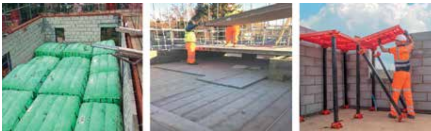
Bagged room pre floor installation vs safety decking (crash decking)
