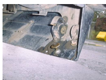
Failed component that caused the incident
