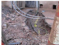
New cable being installed
