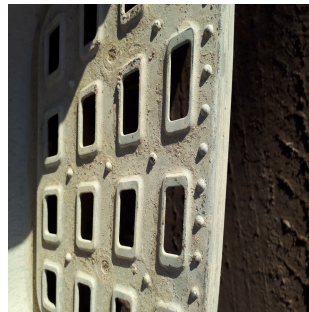
Footplate in good condition
