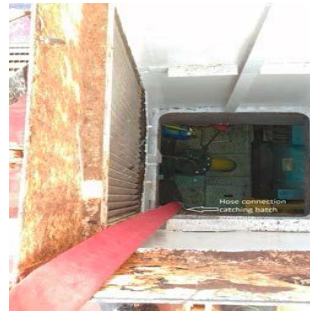
Hatch through which hose was being recovered
