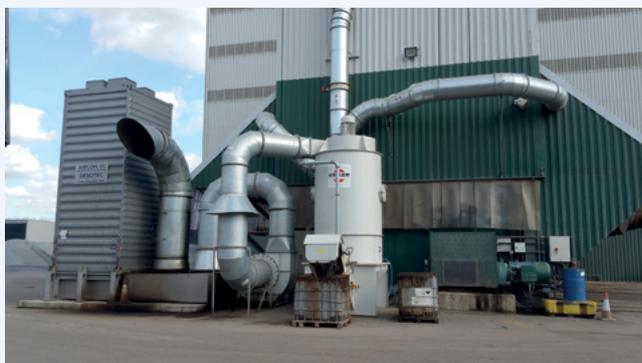
The system extracted fumes and dust from the mixed material storage bins and the vehicle loading bin area. Extractions fans capable of a maximum volume flow of 28,000m<sup>3</sup>/hr were used. The captured emission dust and fumes were processed through a wet scrubber, which removed heavier particles, and then a carbon filtration system to remove nuisance fumes.
