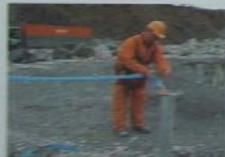
Figure 29: Installing quarry face edge protection
