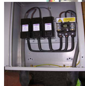
New panel with IP2X protection
