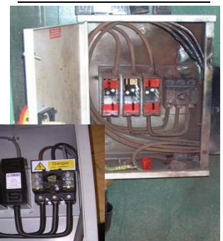
Panel after short circuit
