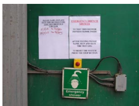
Alarm system for drench showers
