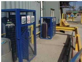
Safer storage of bottled gas
