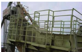
Handrails around the screen deck platform
