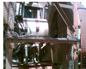
Burner withdrawn for maintenance
