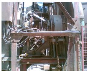
Burner in operation
