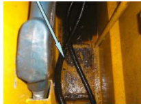
Original battery position with restricted access
