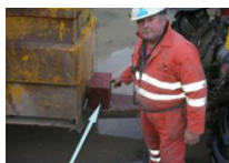
New external battery location
