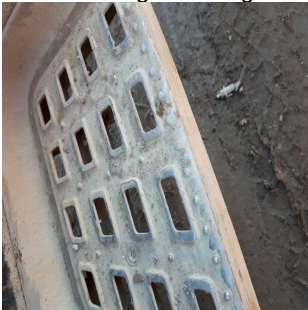
Footplate in poor condition
