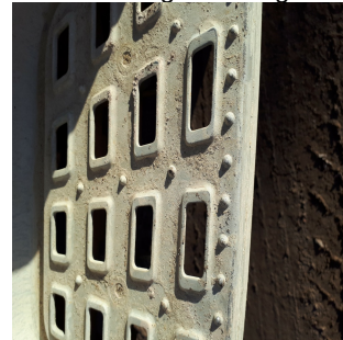
Footplate in good condition
