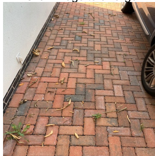
Debris in drive
