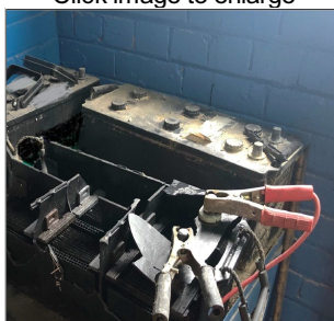
Photograph showing the damage to the battery casing after the explosion. Also shown is an intact battery with its six cell caps fitted.
