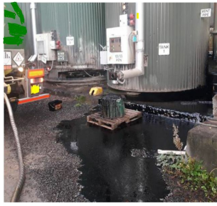
Photograph 1 - Spillage of Material
