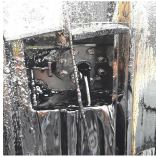
Butterfly Valve with Sensor Probe removed
