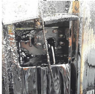
Butterfly Valve with Sensor Probe removed
