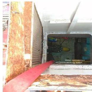
Hatch through which hose was being recovered
