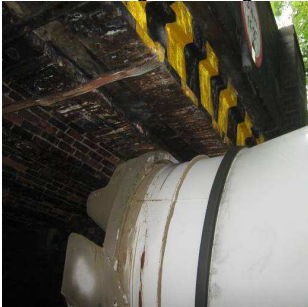
Wedged under Low Bridge
