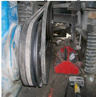
Drive belt that was being worked on
