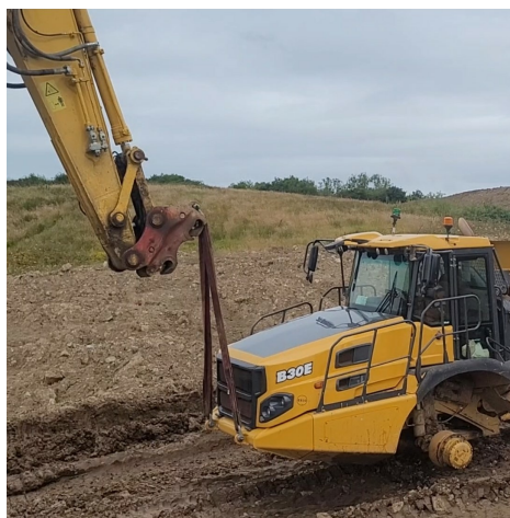
Use of excavator with lifting equipment
