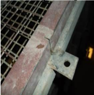
Guarding Being Cut
