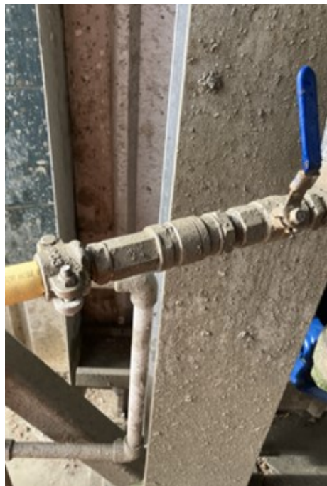
Image above shows a magnetic coupling in place and a typical example of a connection without one.
