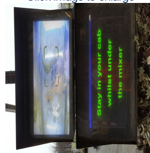
Screens providing info to drivers whilst sitting in cabs
