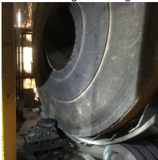
Before - shows access
