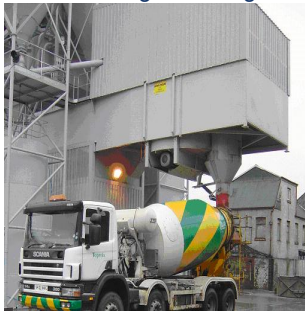
drive through loading point
