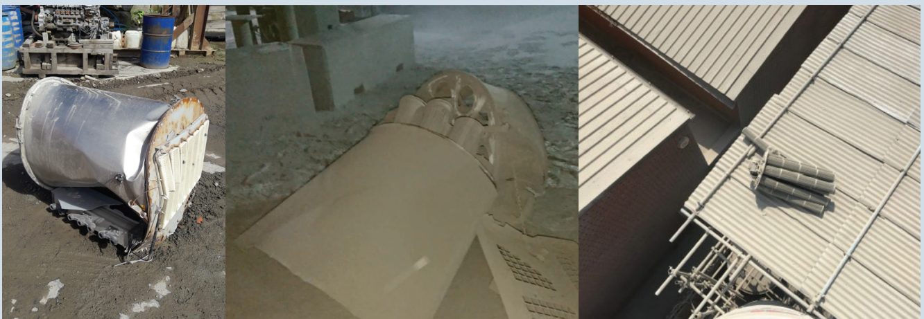
Over-pressurisation incidents lead to the 'launching' of these filter/filter housings from silos. If these had landed on anyone they would have been killed.
