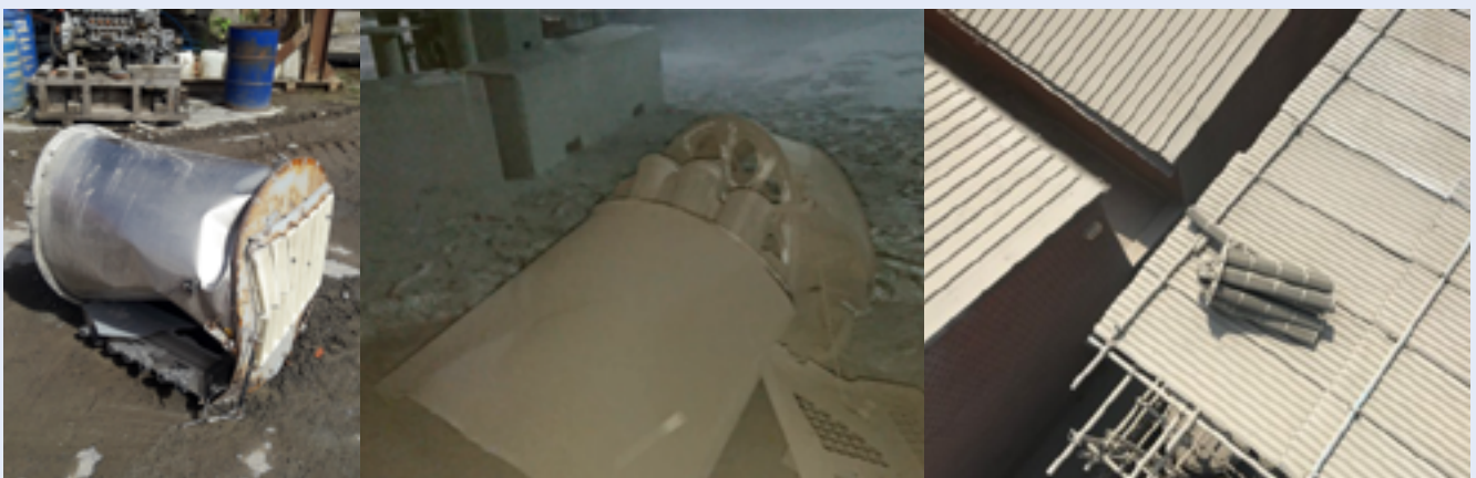
An over-pressurisation incident lead to the 'launching' of this filter housing from the top of a silo. If this had landed on anyone, they would have been killed.
