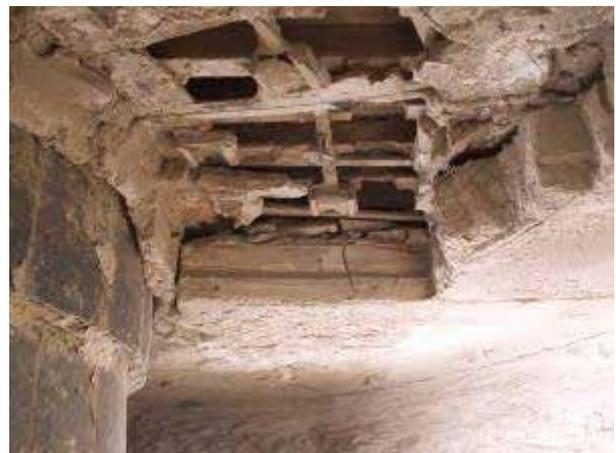
Figure 1: Cyclone roof with partially wrecked refractory
