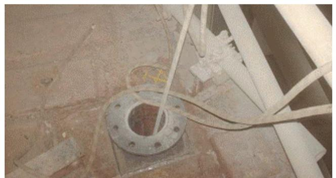
The ropes are then hooked and dragged through access doors
