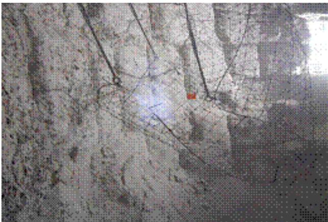
The ropes are pulled out through the cyclone roof, disconnected and the tensioning rods are fitted through the brackets and tensioned.
