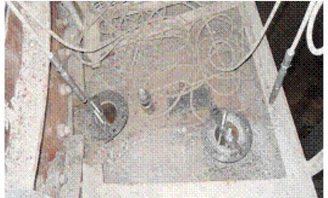
The nets are tensioned and pulled up tight to the underside of the roof and the refractory roof is restrained.
