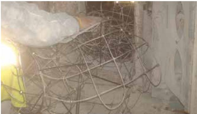
The connected net is then pulled up to the underside of the roof
