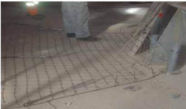
The connected net is then fed back into the cyclone through the access door
