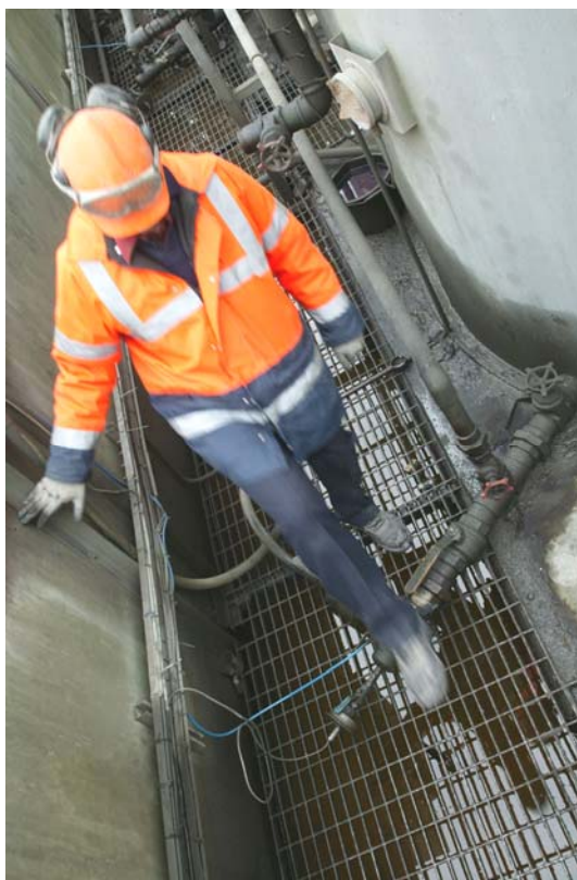
A slip, trip and fall hazard in the cement industry
