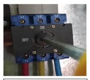
Metal bar that connects the outer isolator switch to the spigot and the contactor on/off switch within the electrical cabinet.
