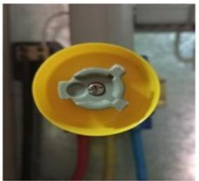
Picture shows the spigot that is attached to both the external isolator switch and the metal bar that is inserted into the contactor within the electrical cabinet.
