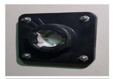
Picture identifies the rear view of the isolator mounted on the inside front panel of the electrical cabinet.
