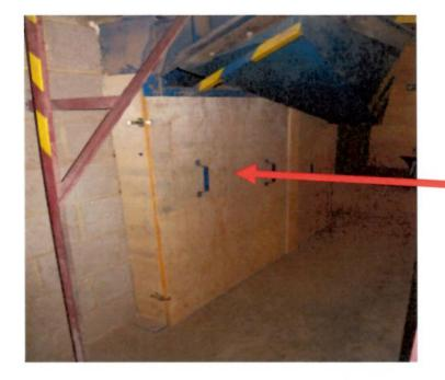
Wooden covers with rubber seals used to prevent dust transferring into working area
