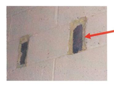
Holes in wall sealed off using expanding foam and bricks
