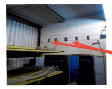
Wall separating Rumbler drum and working area. There were multiple points where dust was able to enter the working area
