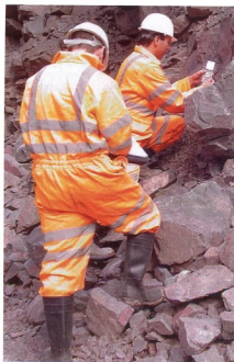
Fig. 5 A potentially unsafe and possibly redundant method of obtaining discontinuity data
