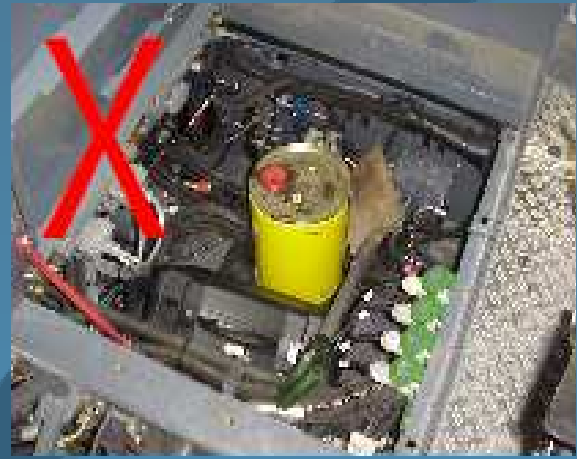
Compartment being used for storage
