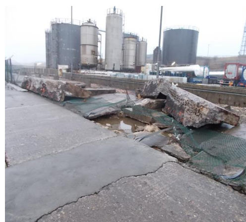
Picture of the damaged wave guard
