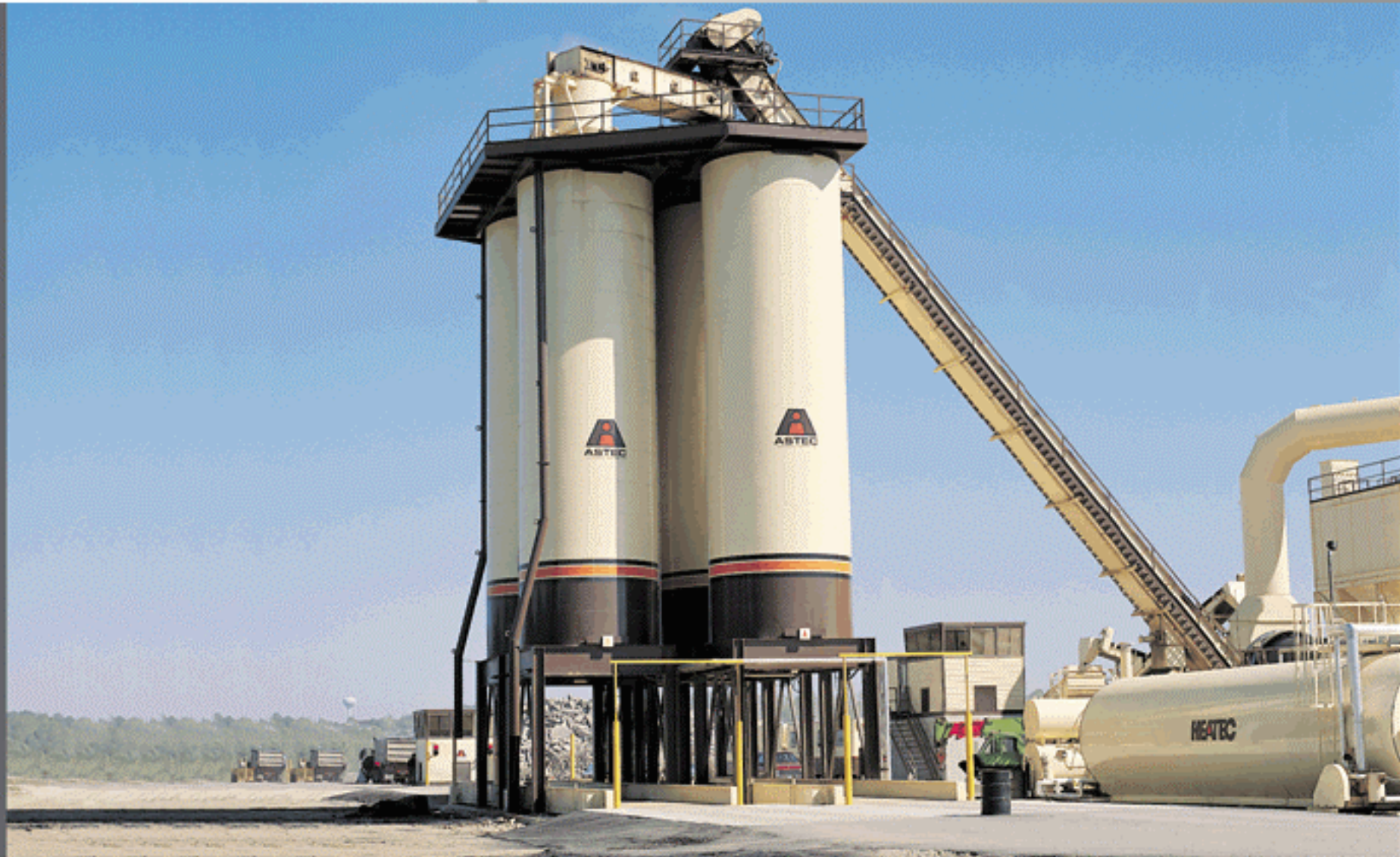
MUTIPLE SILO SYSTEM
