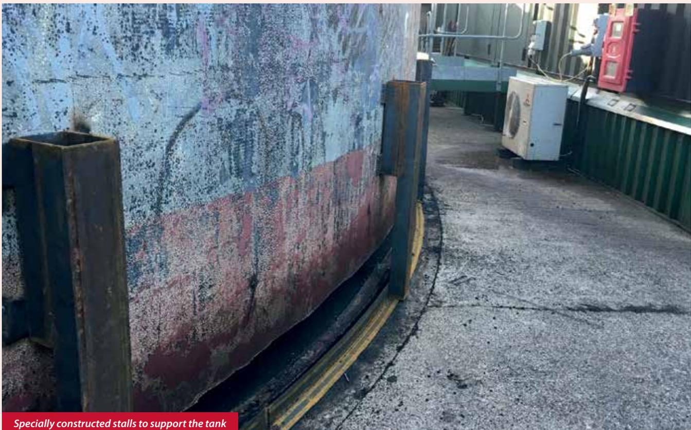
Specially constructed stalls to support the tank
