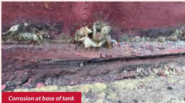
**Corrosion at base of tank**
